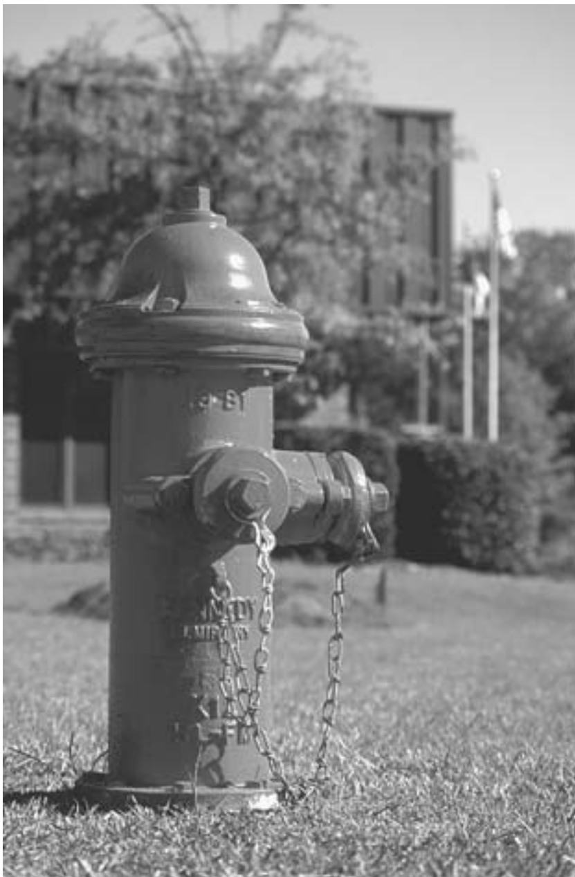
FIGURE 9.8 Barrel-type fire hydrant
