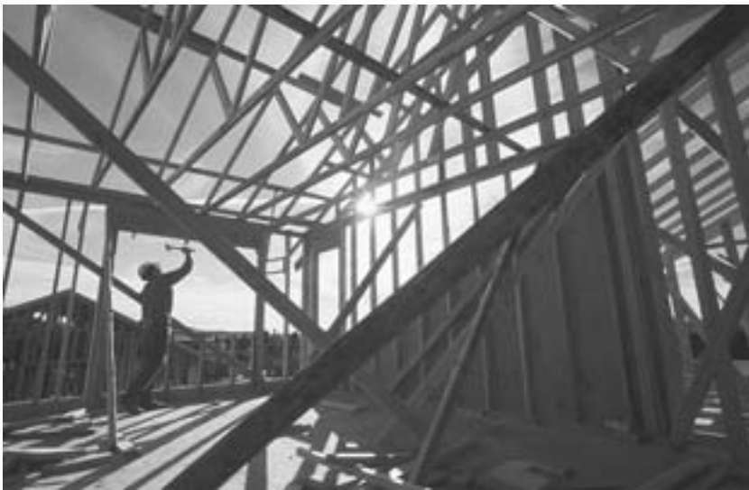
FIGURE 5.2 Wood-frame construction
